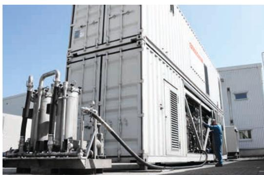
The nitrogen covering means no explosive zone can arise within the gas-tight decanter from FILTRATEC. The three phases of oil, water and solid result in only one step
