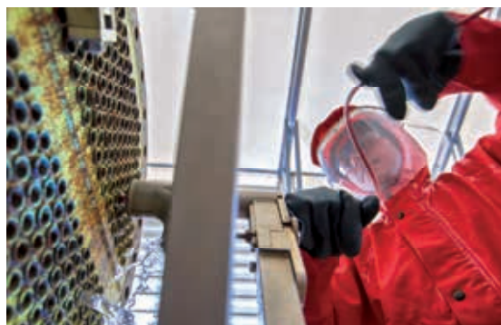
Our UHP jetting equipment is able to remove even the most stubborn coke deposits from heat exchangers
